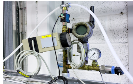
Various types of instruments on UBD-model like valves, wired/wireless pressure transmitter and flow transmitter
