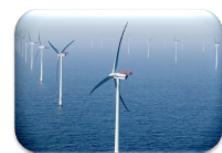
Power Generation Systems
